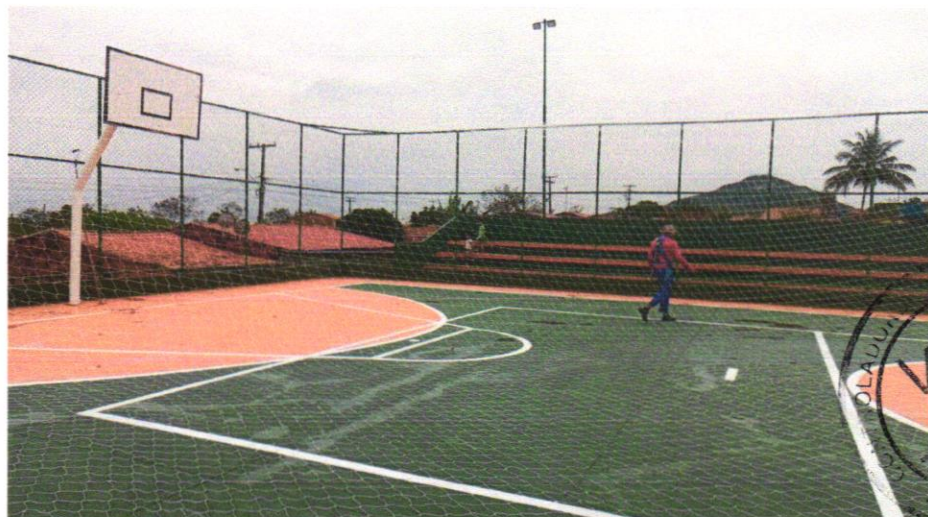
Foto 06 - Tela de nylon, fio 30-36 (3,6mm), malha 10x10cm
